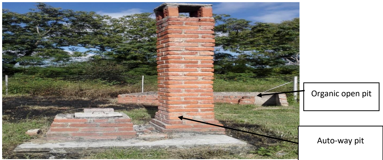
Plate 2: Auto-way pit and organic open pit used to dispose pathological waste and organic waste respectively at STT hospital.
