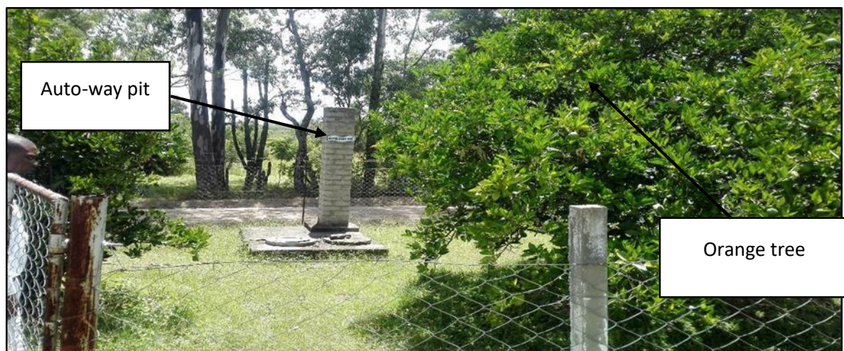
Fig. 18: Auto-way pit (located in a minor orchard) used to dispose pathological waste at Holy Cross hospital.
