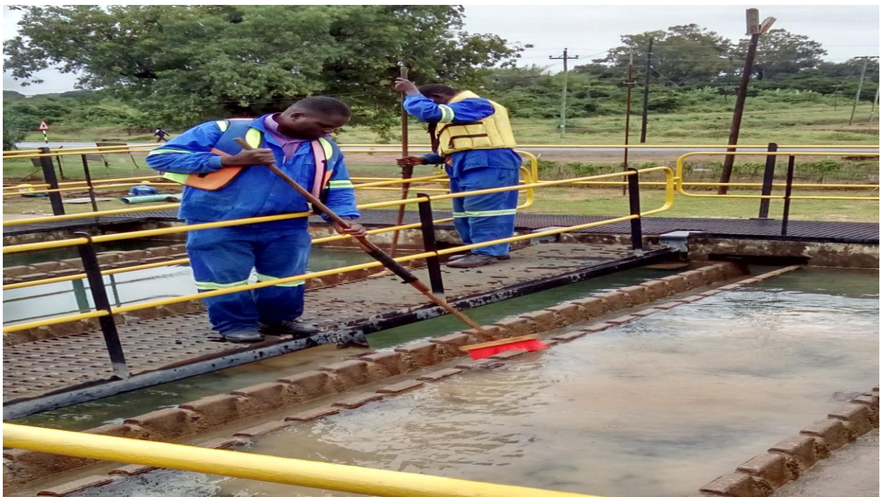
Plate 10 ( Workers cleaning the filters at Chiredzi water treatment plant (CWTP). )
