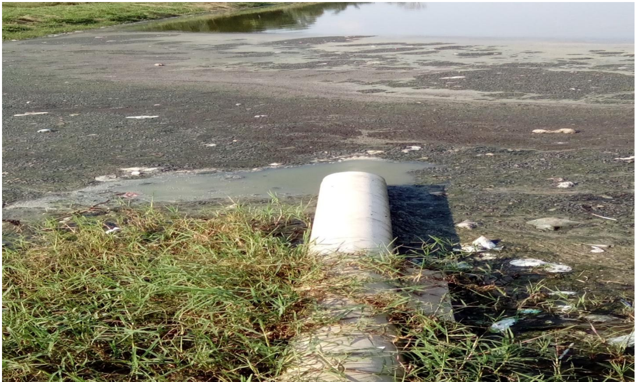
Plate 11 ( One of the wastewater ponds, showing poor management in CTC )
