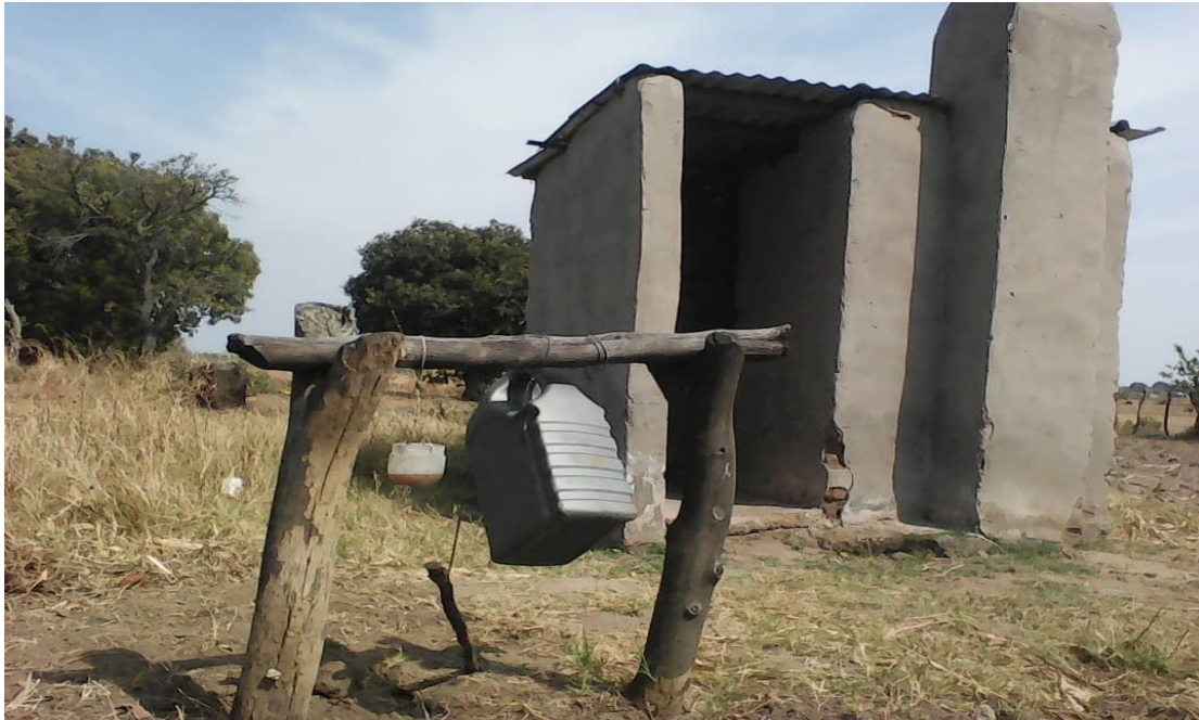
Fig 2: showing evidence of wash program on toilet construction
