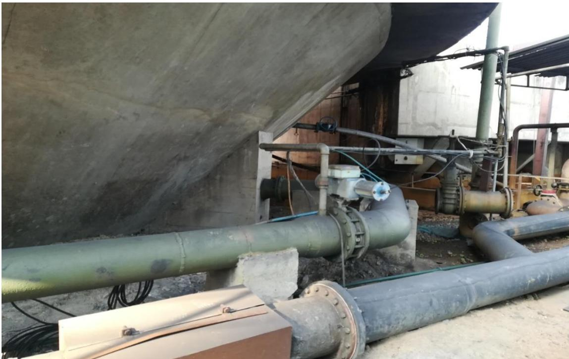
**Figure 2.3 Bottom of the clarifier and the clarifier inlet valve**
