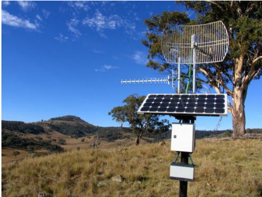
Figure 29 Complete installation setup [20]
