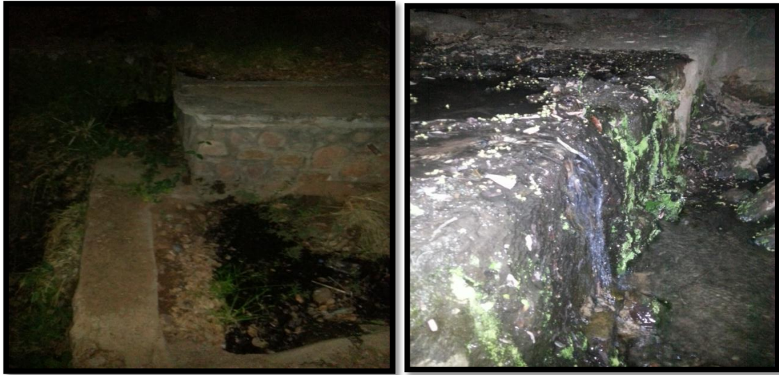
Figure4. 5a Shows a well built structure that captures pressurized water from the ground to the irrigation and to taps. While figure 4.5b shows water that has escaped from the capture tank. This place has similar function as the Masibinta springs.
