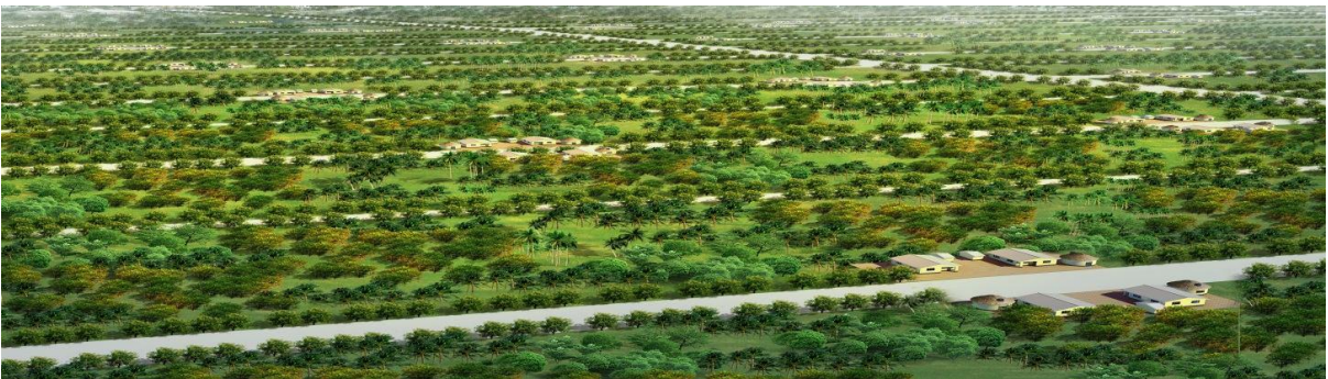
Fig 7 below shows Odzi relocation area site view showing houses, schools, clinic and roads
