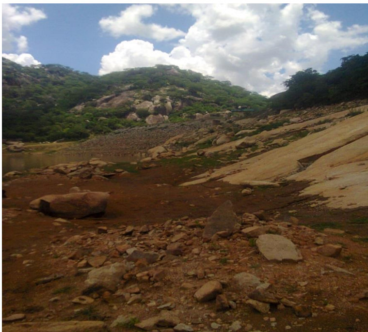
Figure 3 shows current water levels on the dam wall of Siya dam
